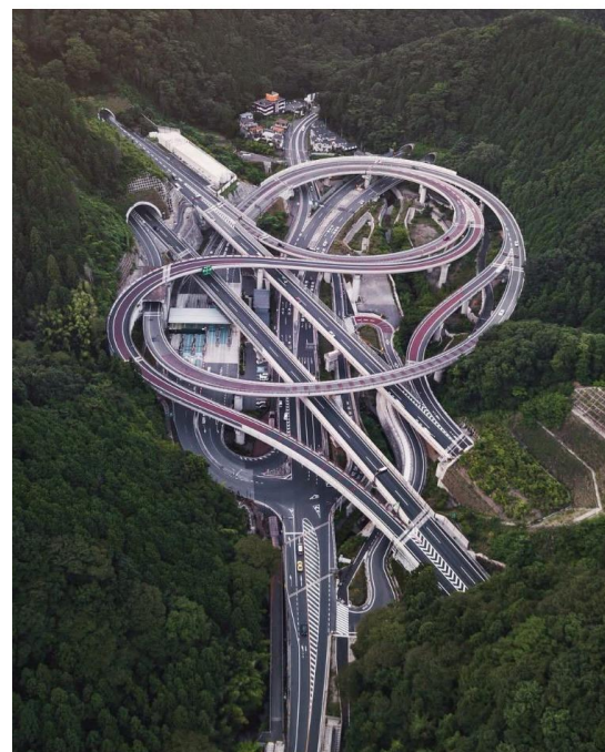
Hisashimichi interchange situated in Hachioji, near Tokyo, Japan 🇯🇵
